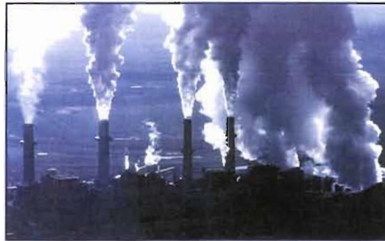
Four-Corners power plant
