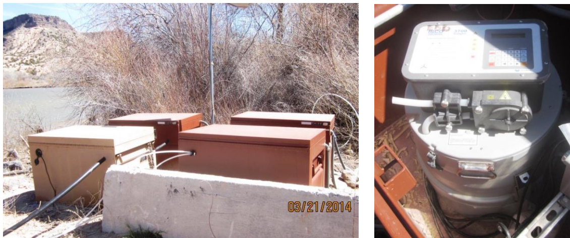
Figure 8. BDD intake station set up.
