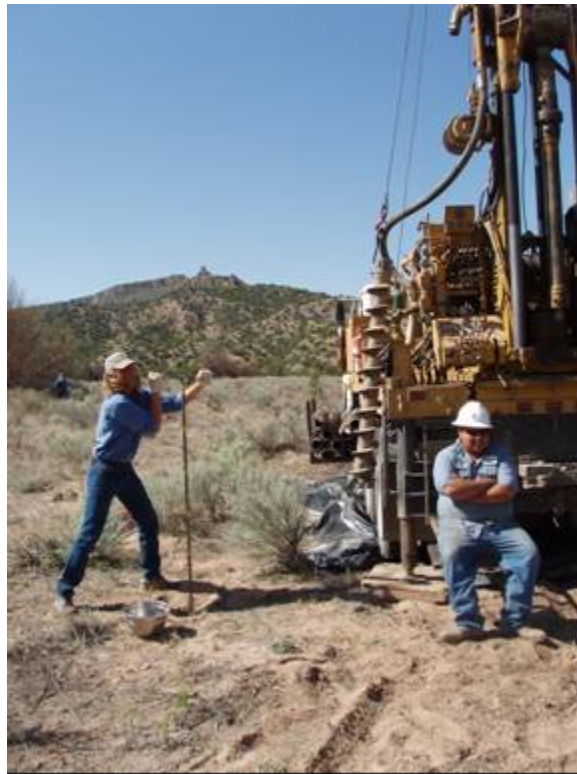
Figure 3. Hand augur operation and hollow stem drill rig
