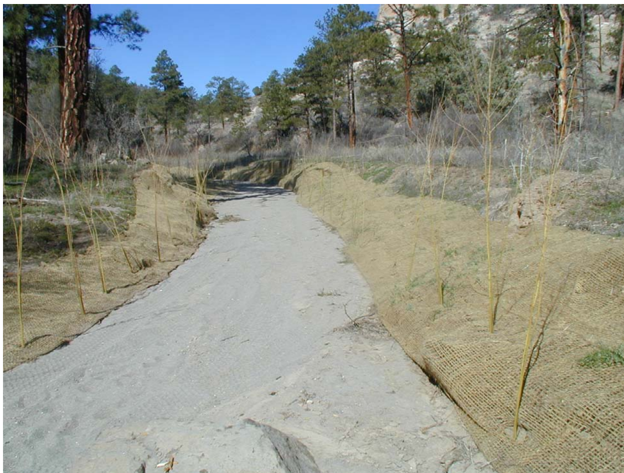
Figure 4.5-1 Photograph of jute mats and willows ( Salix spp. ) used to stabilize banks in Pueblo Canyon, spring 2005 (view to the west)
