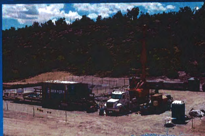
A crew drilled CrEx-1, the project's first extraction well for hydraulic control.
