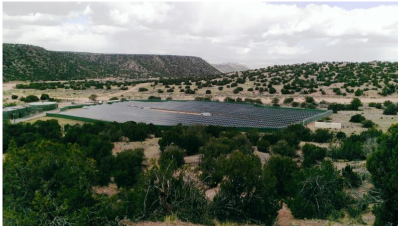
The Buckman Direct Diversion 2A Solar Field
