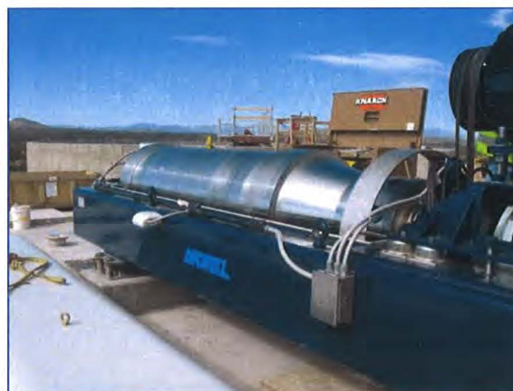
Figure 9: Dewatering Centrifuges at BDD during Installation
