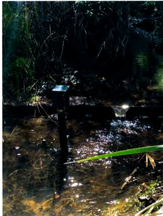
Figure 13. Equipped Stilling Well B, looking upstream along the Bypass Channel, July 26, 2018
