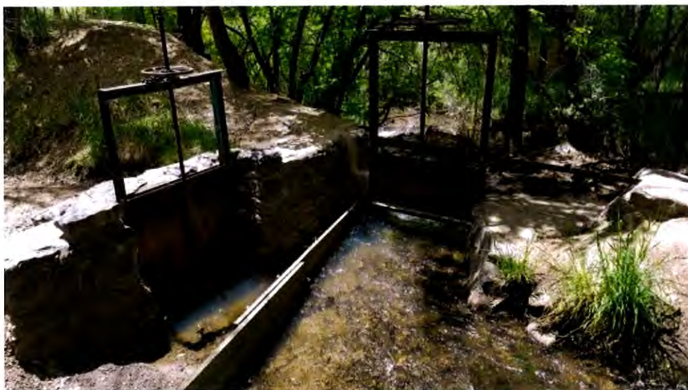
Figure 25. Acequia Madre headgate (closed) on left, and headgate to the Santa Fe River on right 5/18/17
