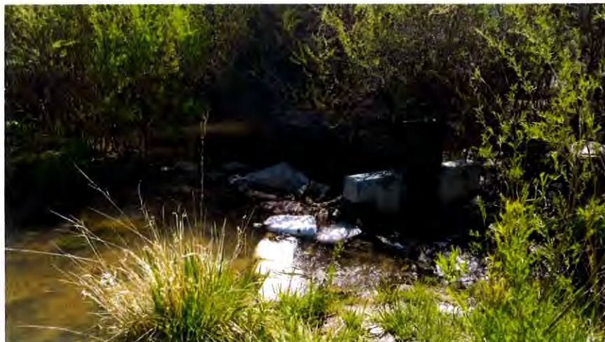
Figure 11. Headgate at TNC Diversion (The Nature Conservancy diversion on the left, and Santa Fe River bypass channel on the right), looking upstream, 5/18/17
