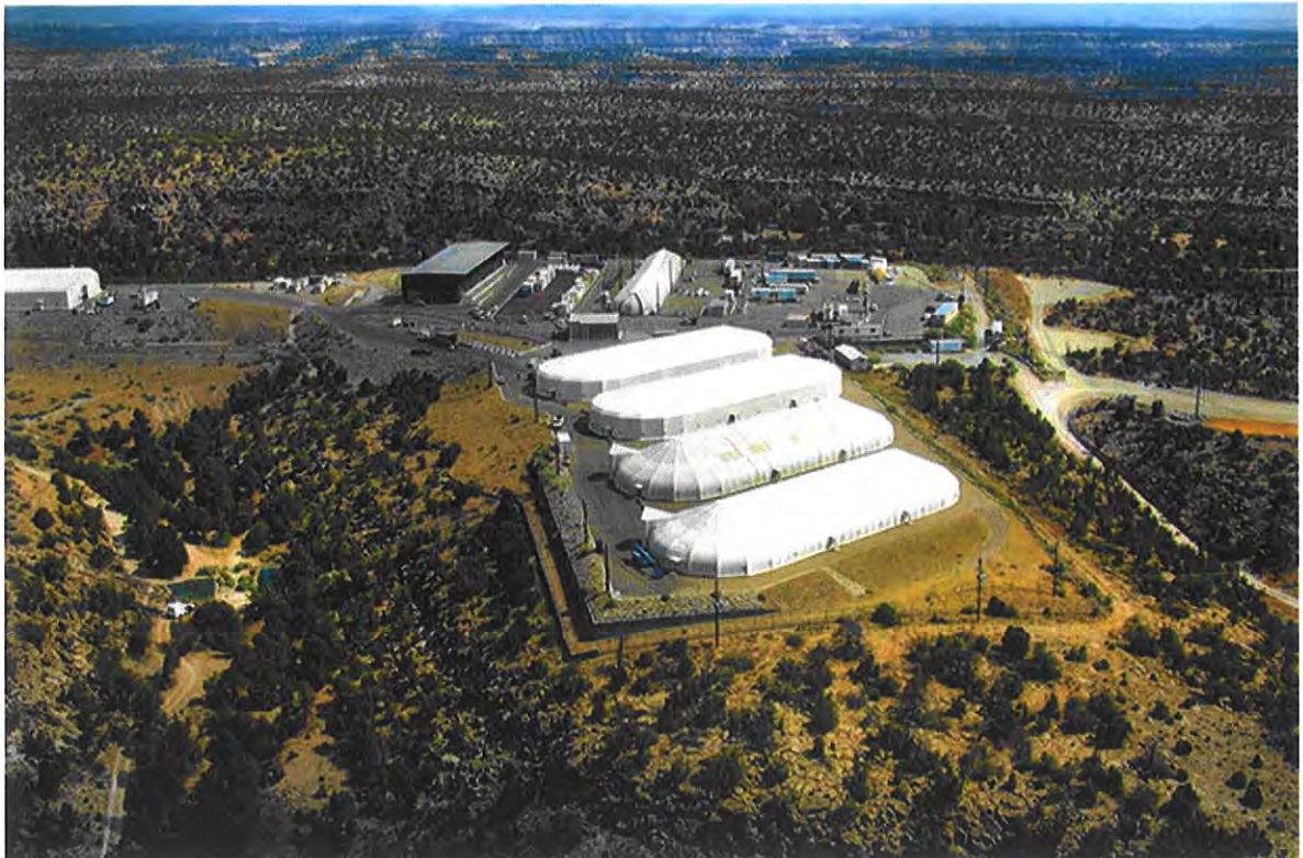
Area G, the legacy waste storage area at Los Alamos National Labs. US DEPARTMENT OF ENERGY
