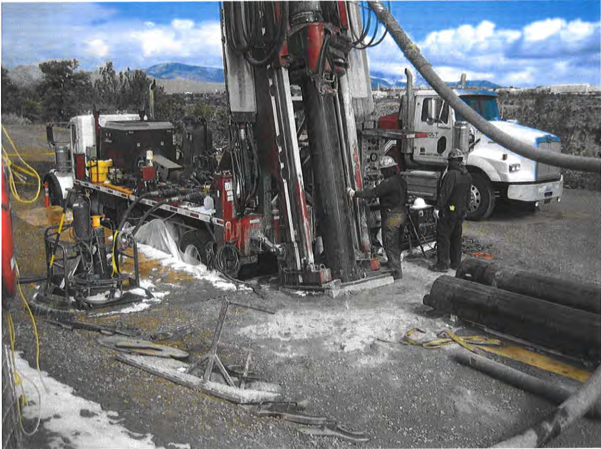
This March 2016 photo provided by Los Alamos National Laboratory shows an angled injection well ...
