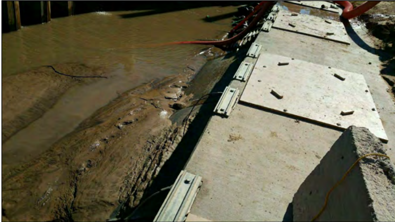
Figure 25. Photograph from April 2015 Inspection Showing Excessive Sediment on Screens
